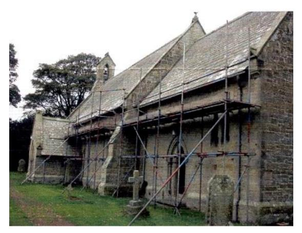
New soffit boards were installed and the area under the eaves was painted.
