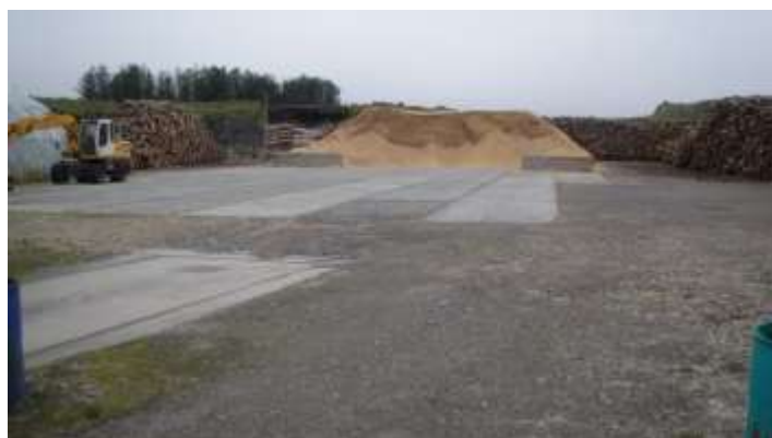
Figure 5: Ingis Biomass store of logs and wood chips in Borrowstone Quarry
