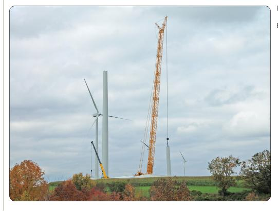
Photo 12 Erection of turbine
