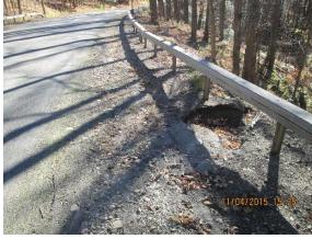
DETERIORATED AND WASHED OUT WEST SHOULDER
