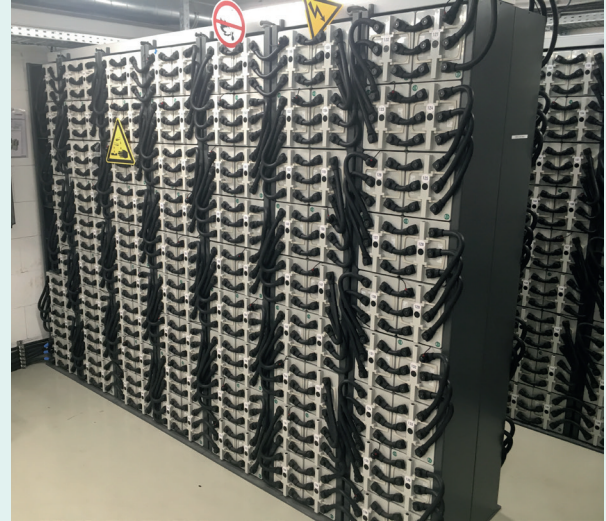
2 x 240 600 Ah; 2 x 288 kWh nominal; Rack size (L x W x H) 2 x 3018 x 662 x 2107 in mm
